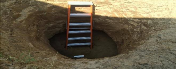
Fig. 8. Identify the distance and put the cable inside the whole process.
